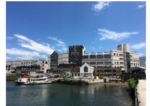
Coaska Bayside Stores
